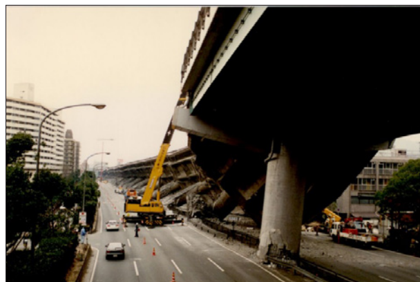
FIGURE 2 Collapse of Hanshin Expressway elevated highway bridge during the 1995 earthquake in Kobe, Japan. Photo by C. Rojahn.
